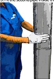
This way you can assemble required number of MKS system elements. The system allows for the use of securing clamps stabilizing the chimney. Method for assembly of clamps is presented in assembly instructions for the MKD system.
